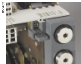
056452 Racking interlock
